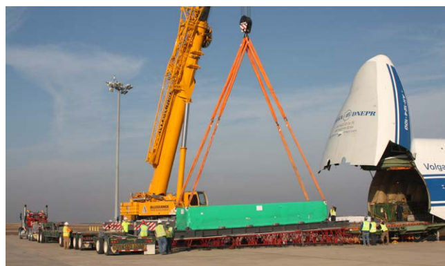
The plate bundle is offloaded from the transport airplane at Houston airport
