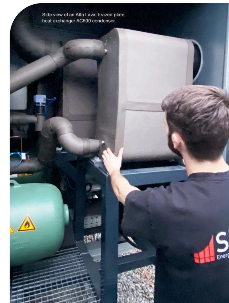
Side view of an Alfa Laval brazed plate heat exchanger AC500 condenser.
