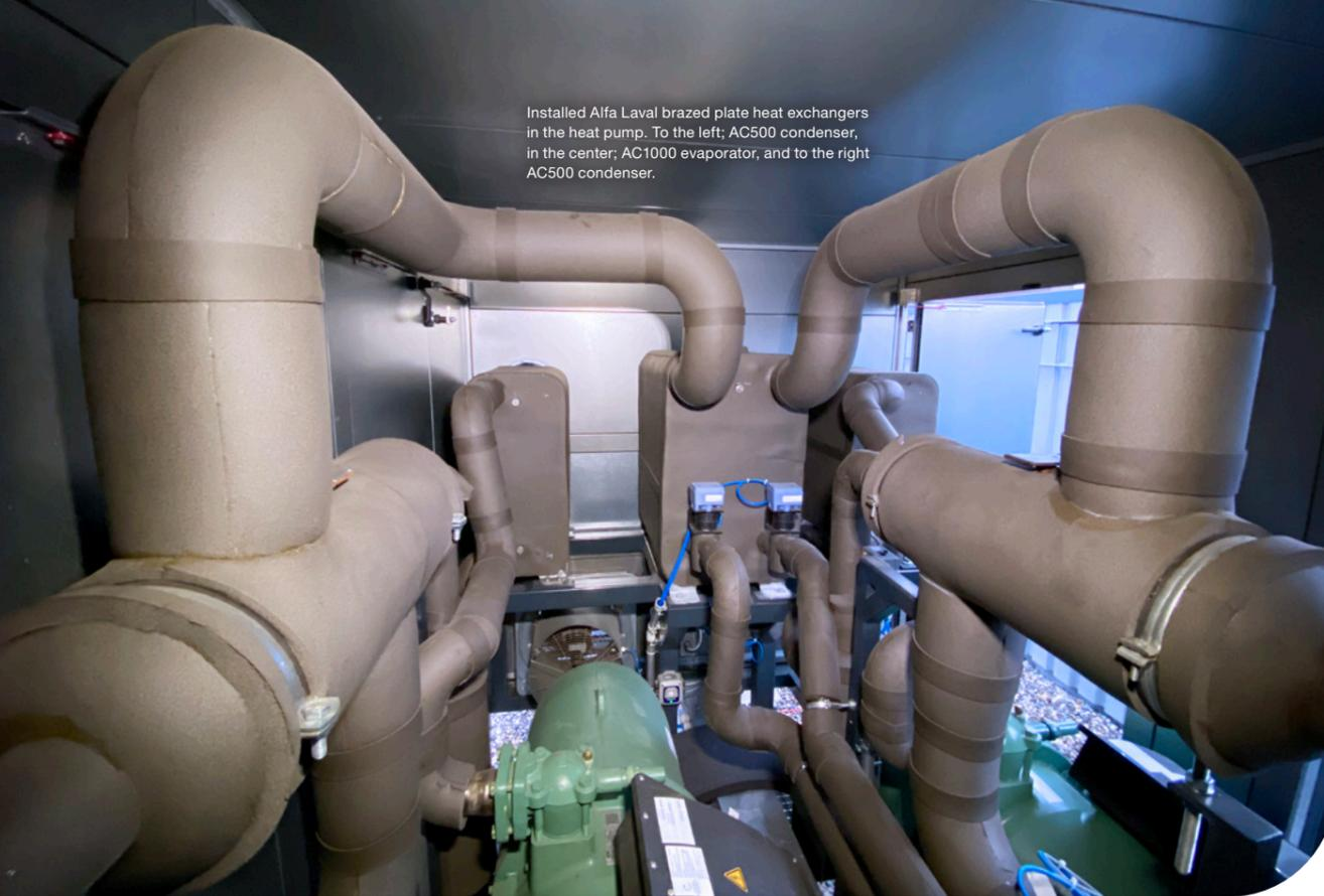
Installed Alfa Laval brazed plate heat exchangers in the heat pump. To the left; AC500 condenser, in the center; AC1000 evaporator, and to the right AC500 condenser.
