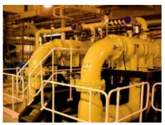
The Alfa Laval ALF filters are mounted horizontally in the seawater piping system.
