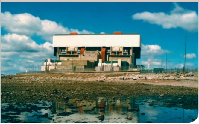
Heysham II is a nuclear power station owned and operated by British Energy, and located just outside the port of Heysham. The plant's two advanced gas-cooled reactors (AGRs) provide steam to two 660 MW steam turbines.
