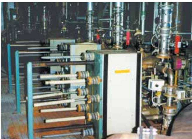
Three of twelve Diabon F100 plate heat exchangers installed at Outokumpu Polarit for temperature control of the pickling lines.
