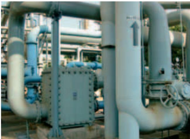
Kakogawa plant. Sulphur is removed in a conventional absorption/stripping system, and the Compabloc units are used to cool the absorbent before it enters the absorption tower.
