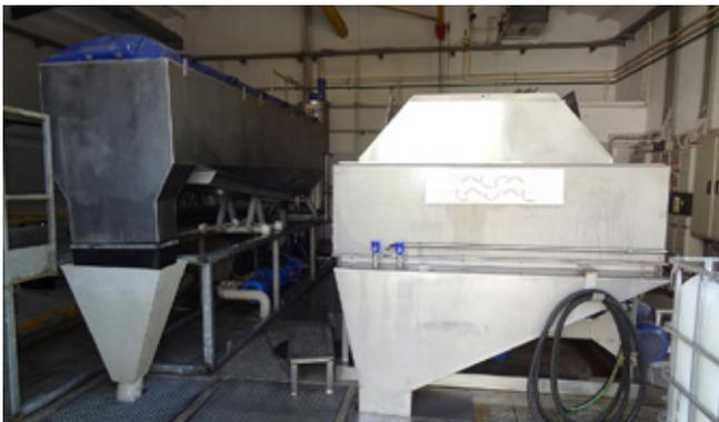
The existing rotating Alfa Laval Drum Thickener (left) and the new Alfa Laval AS-H Belt Thickener.
