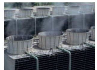
... cooling towers, irrigation etc.
